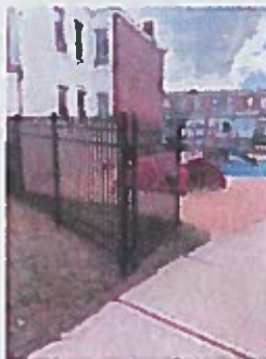
New Bromley Center fence through CDBG grant
